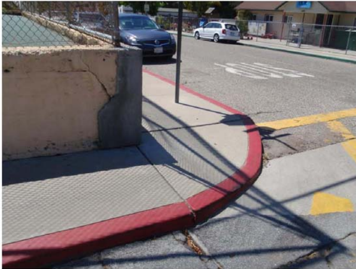
Curb ramp at Wadsworth and Bello Avenues
