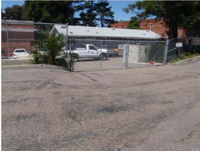
Asphalt ramp and temporary building at rear of project
