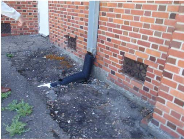
Downspout on northerly side of building
