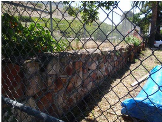
Retaining wall at rear of property
