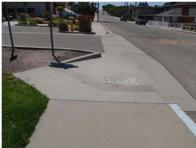
Curb ramp at police station driveway
